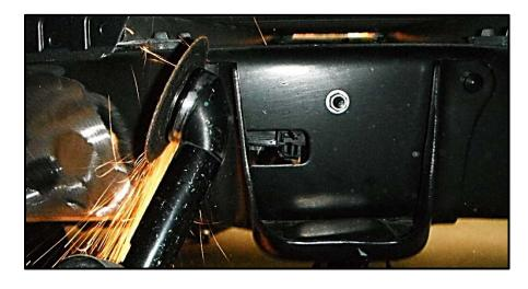
2. Remove the 4 rivets holding the stock bump stop mount on frame. A disc cutter and air chisel/air hammer will be needed to remove rivets. Using the disc cutter, cut an X through the head of each rivet. Use the air chisel to knock each piece of the rivet head off. Remove the bracket and sand the remaining part of the rivet flush with the frame. Drill a small hole in the center of each rivet and use
