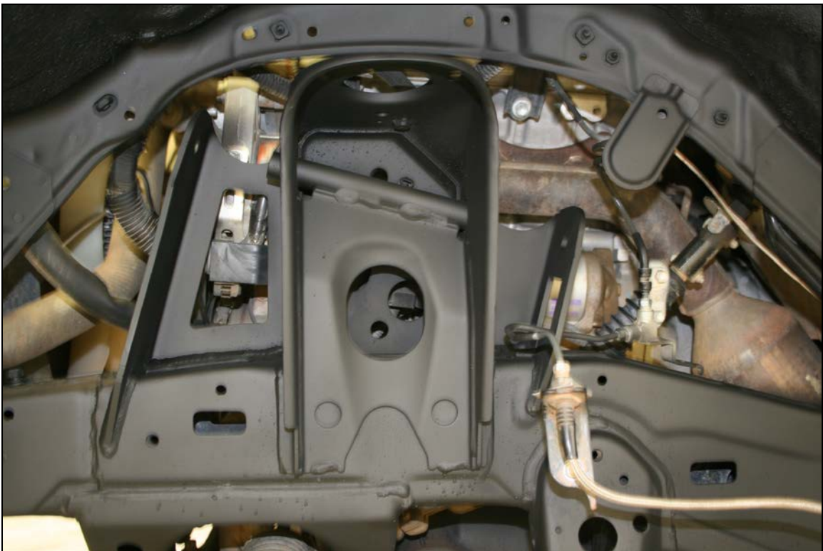
(2-2) Gussets welded and painted.
